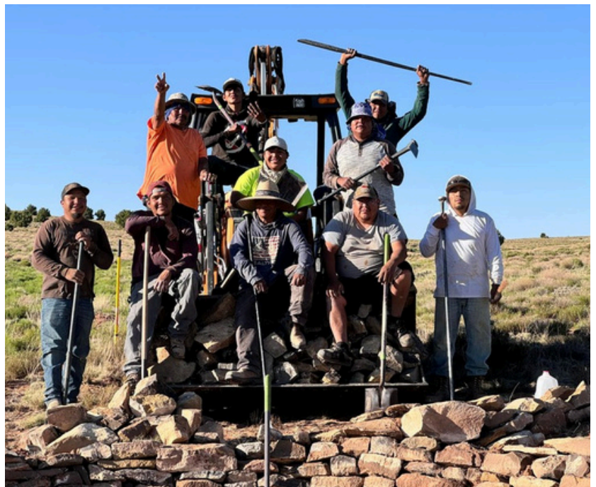
Constructing water catchment systems in corn fields; Nihikeya
